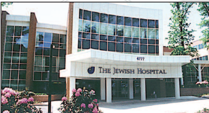
Administrators at Cincinnati's Jewish Hospital are especially impressed with the quality of Masterplan's employee training programs.
